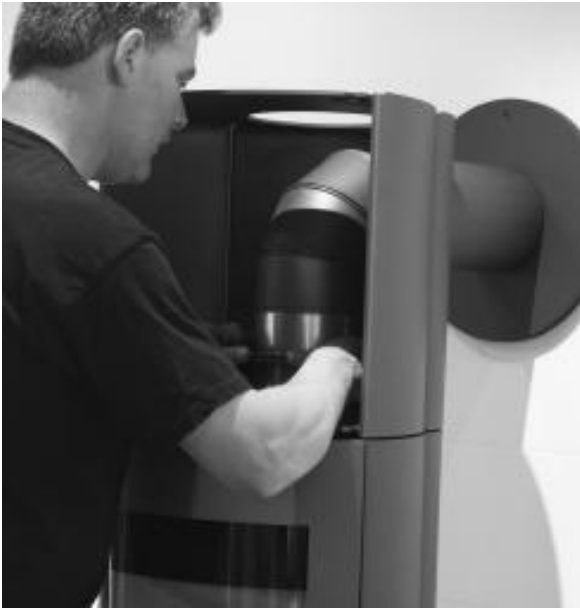
5. Installing the flue for rear outlet Secure the wall plate (if applicable). Connect the flue pipe
