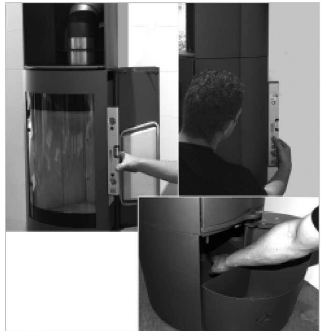
8. Levelling Open the small door in the base. Use the adjusting feet to level the stove. Position the level as shown in the picture.
