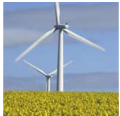
THE EVERHOT IS PARTICULARLY SUITABLE FOR SUSTAINABLE ENERGY PROJECTS
