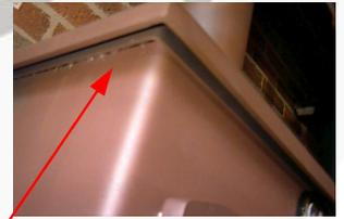
Check the rope seal there should be an even width of exposed rope all the way around the under side of the top.
