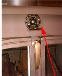
The optional stove thermometer shows the temperature the stove is operating at. It should always be above 300 °f But not above 600 °f.
