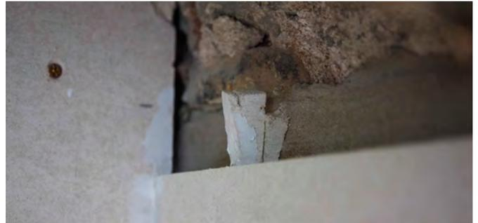
Using a PROMAFOUR® wedge to correct uneven walls.
